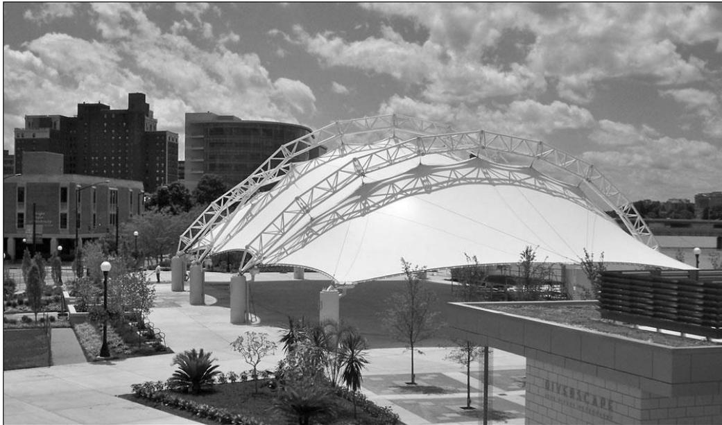
**Figure 1.** Tensioned Fabric Structure
